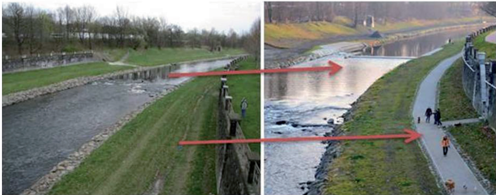
Fig. 3: Weirs with the fish passage under the bridge Sýkora, walking trails and multi-purpose communication.
