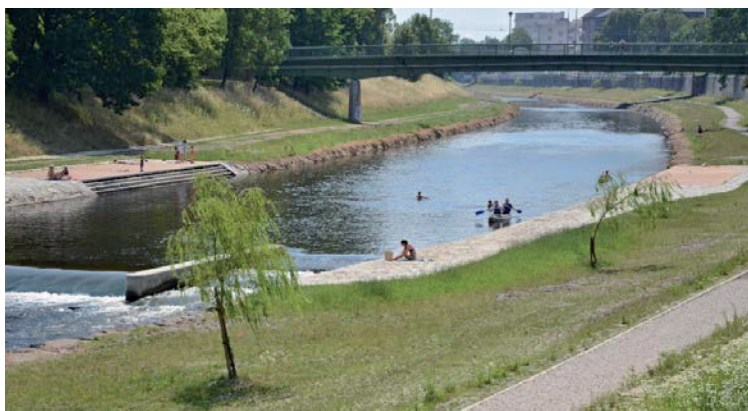
Fig. 1: Restoration modifications of the model locality – Ostravice river in the center of Ostrava.
